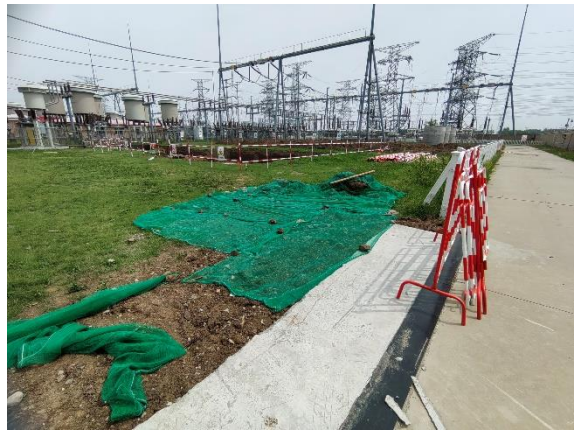
蒲河变电临时苫盖
