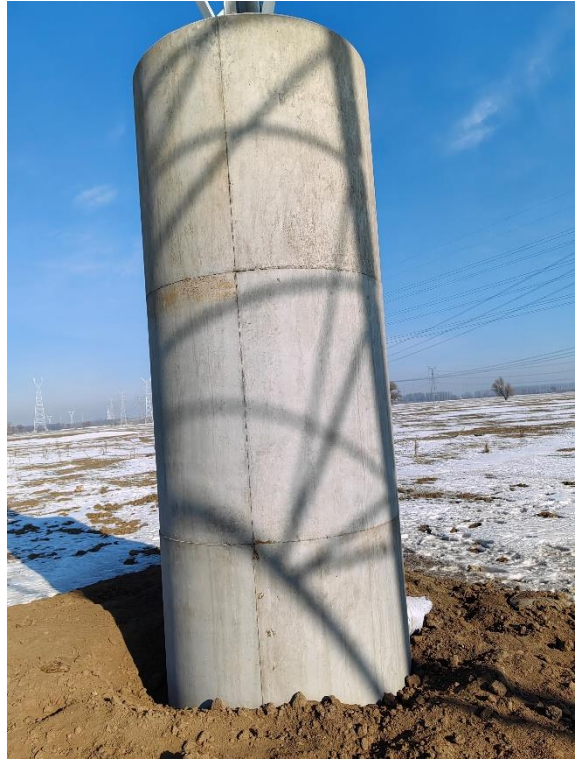
跨辽河塔基基础
